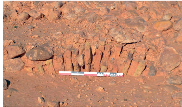
Fig. 5 - The upper part of one of the arches in the stretch built on arcuationes (photo by author).
