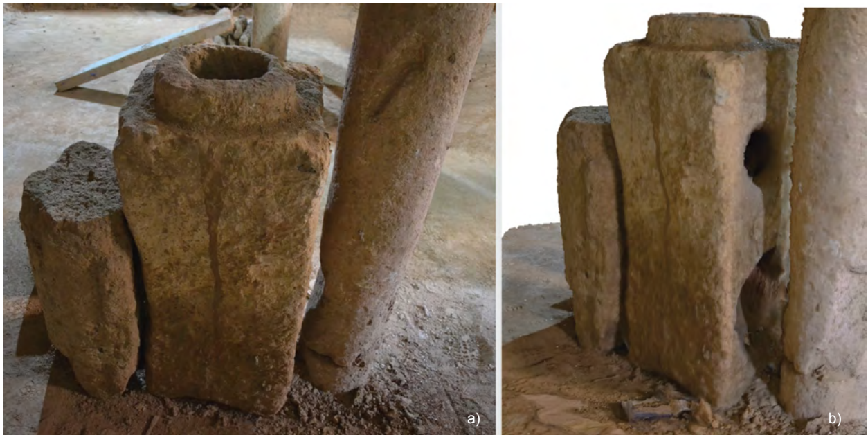
Fig. 6 - a) the lithic pipe found during the restauration work of the Venerable Marabout Sidi Moussa El Akkdahari, Biskra; b) 3D model of the lithic pipe: view of the two holes on the side (courtesy by Luigi Magnini).
